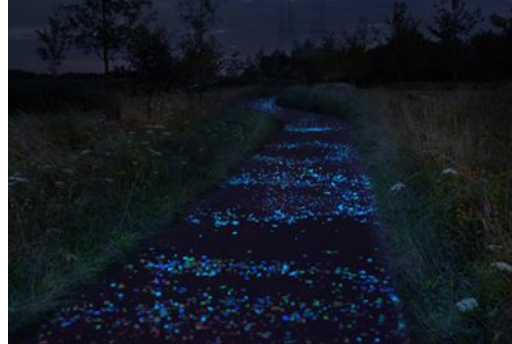
Figure 6.6 'van Gogh' cycling road, enlightened by thousands of 'glow in the dark' stones, taking up light in the day and emitting this light during the night (source: www.cultuurgids.avro.nl )
