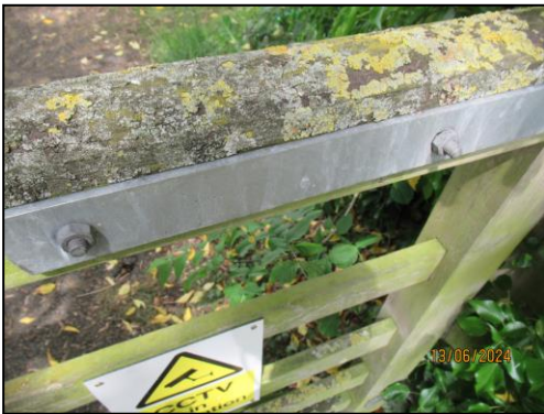
(Excess bolt thread at gate to skate park)
