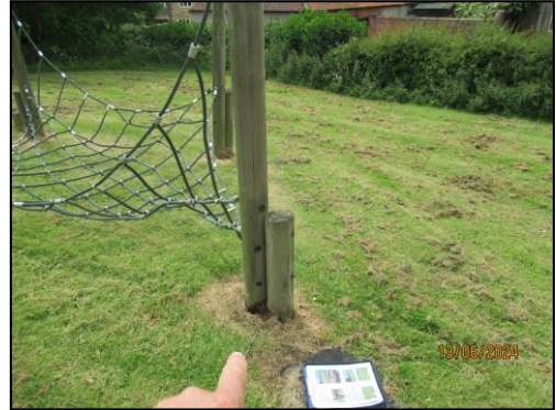
(Location of rotten post on net climber)
