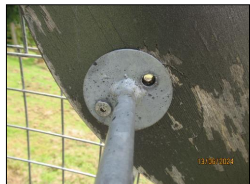
(Missing bolts on back board)
