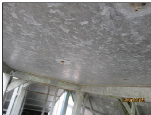
(Protruding rivets)
