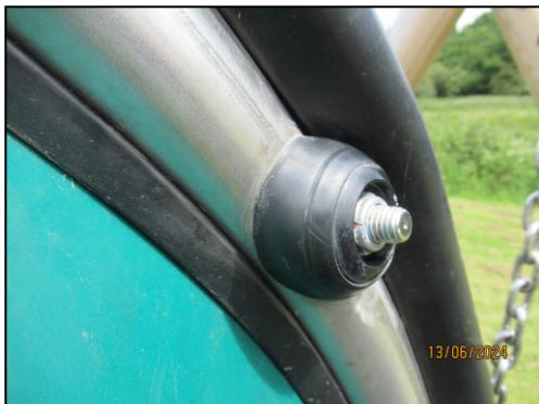
(Missing bolt cover caps beneath seat)
