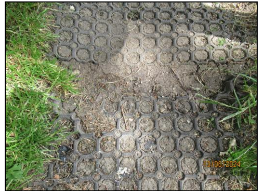
(Damaged grass mat)
