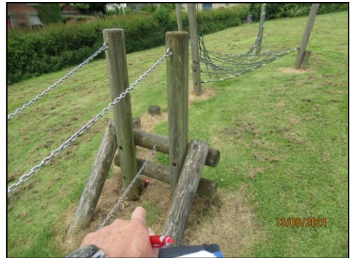
(Rotten post on Burma bridge)
