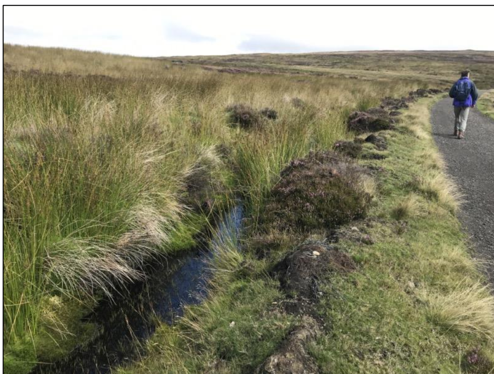
Figure 3-14: Smaller drainage ditches parallel to railway embankment which could be blocked to create pool features
