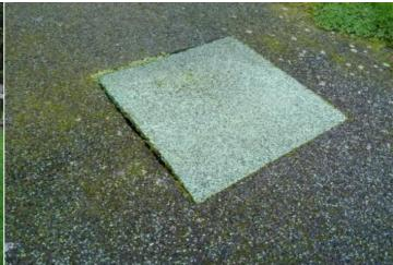
**Finding:** One coloured section is shrinking away from main **Action:** Cut back entire section and infill - 0.75m x 0.75m base and slightly lifting
