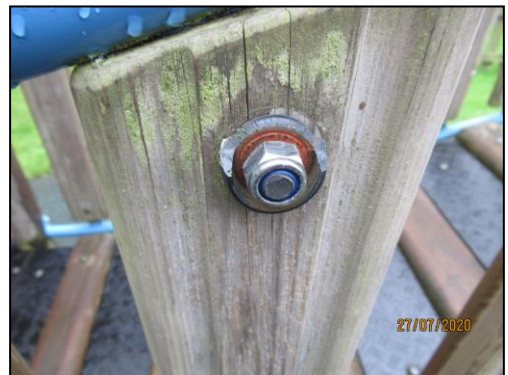
(Broken bolt cover cap)
