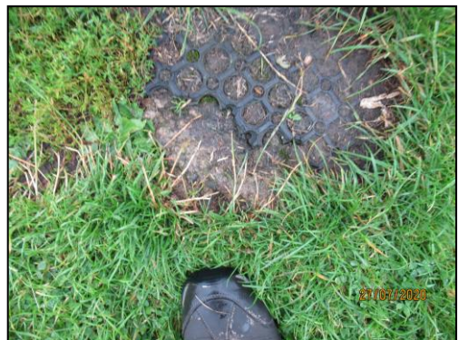
(Exposed foundations at damaged grass mat)
