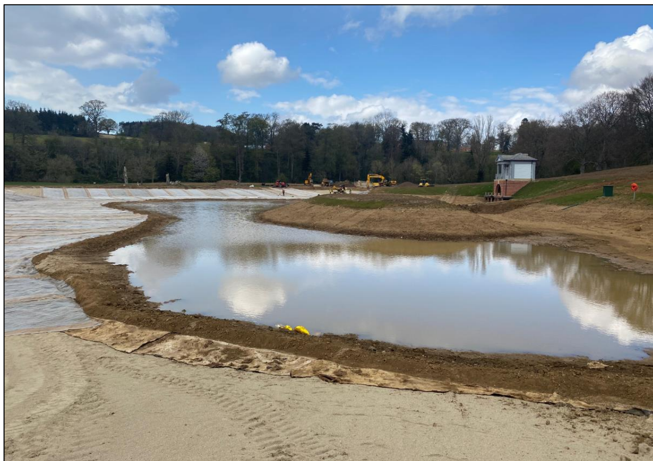
Figure 2-1: Work in progress, showing the lowered floodplain levels of the new lake (May 2021)
