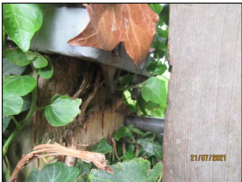
(Gate catch missing stopper)
