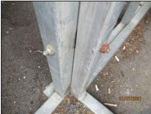
(Excess bolt thread at half pipe)
