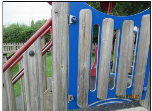
(Broken bolt cover cap)
