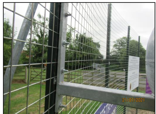
(Excess bolt thread)
