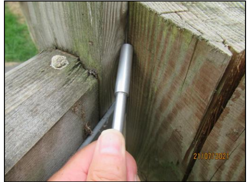
(Potential pinching/crushing hazard at gate at skate park)
