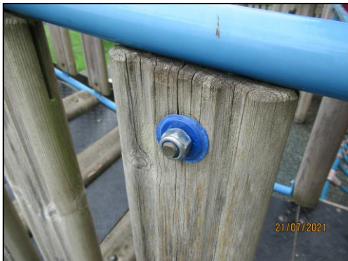
(Broken bolt cover cap)
