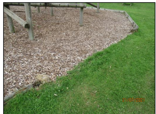
(Missing wood chipping retaining logs)
