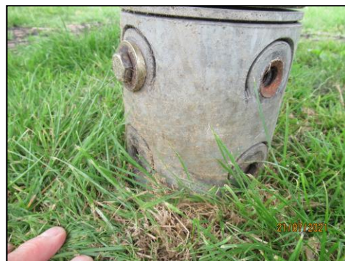
Broken studs at ground fixing
