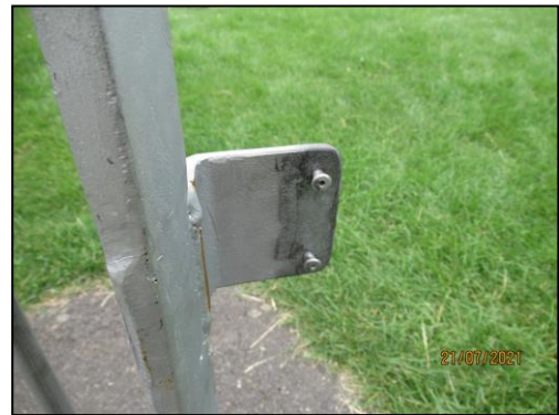
(Missing buffer on gate)
