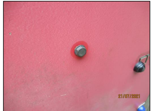
(Broken bolt cover cap)
