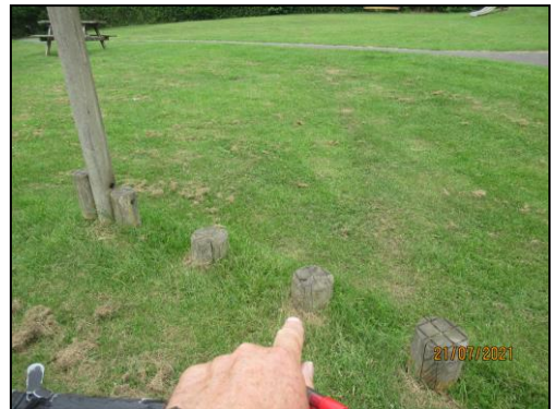
(Location of rotten step post)
