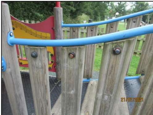
(Broken bolt cover cap)
