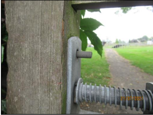
(Missing nut on bolt at gate)
