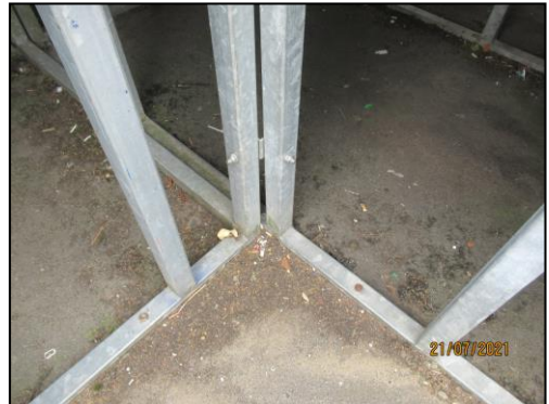
(Excess bolt thread at half pipe)
