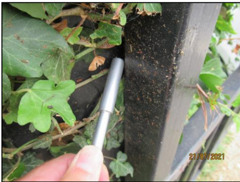
(Potential pinching/crushing hazard at gate to main area)
