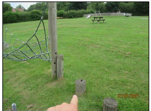
(Location of rotten step post)
