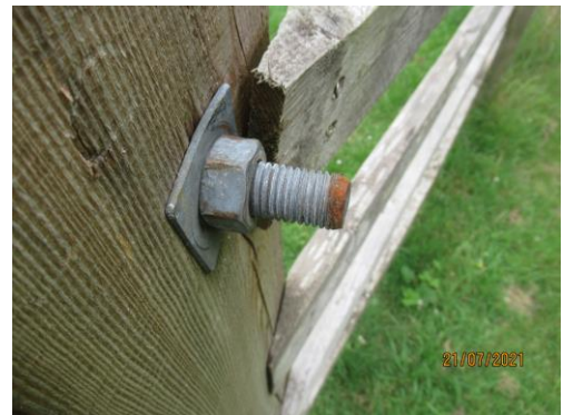
(Excess bolt thread at gate)
