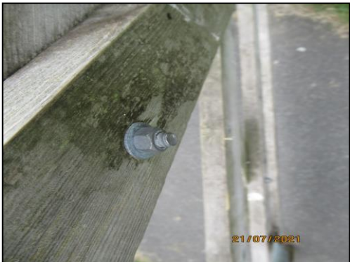
(Excess bolt thread at gate)
