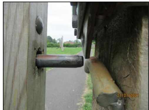
(Gate catch missing stopper)
