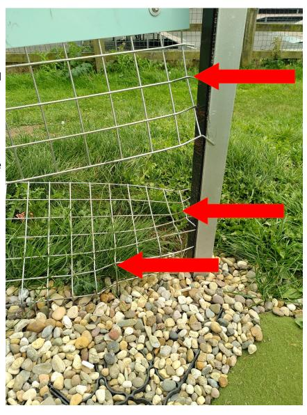
Bottom mesh section has been kicked repeatedly breaking the galvanised mesh clips on 2 side, severing the panel from the fence.
